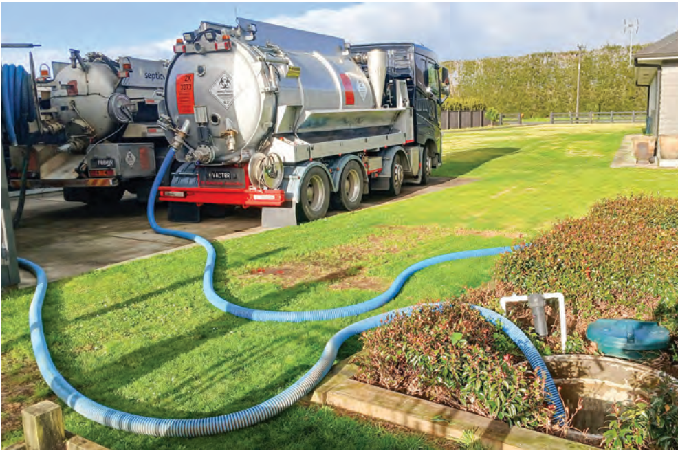
The Septicworks team get to work.
